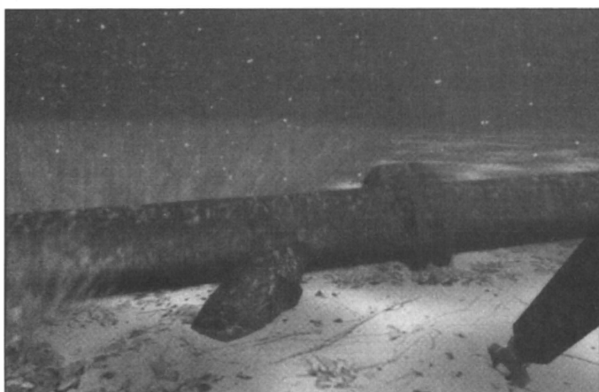
Fig. 6. Fish and particles can generate problems in vision tasks
